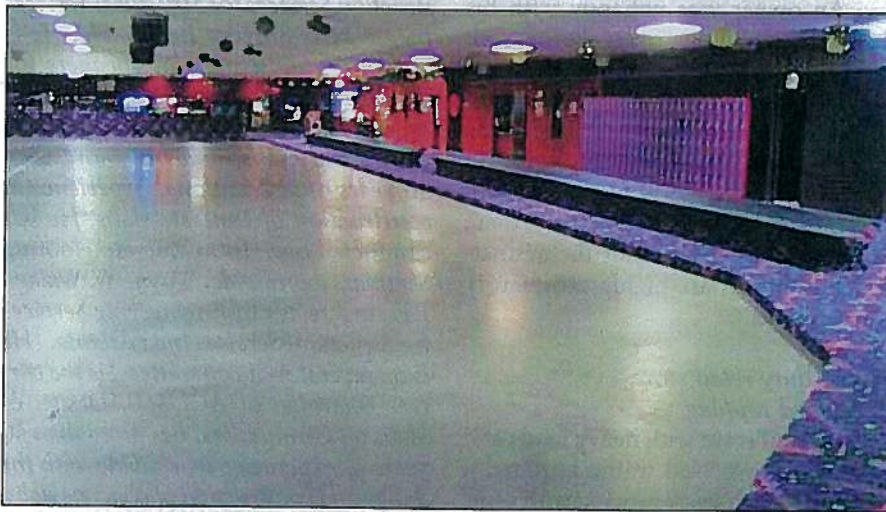
Top: One of four 90x30-foot industrial facility experimental floor slabs. After eight years, only cracked slab had shortest fibers with lowest dosage. Photo: Bob Grace Bottom: 168x84-foot roller skating rink unbonded 4-inch topping slab and no joints or cracks after more than four years. Photo: Tom Baggett
